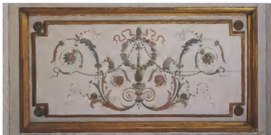
One of the four dado panels that are located below the angled mirrors in the corridors of the Crillon room
